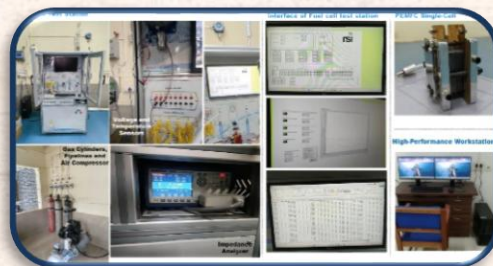
Hydrogen Fuel Cell and Electrolyser Lab (A)
